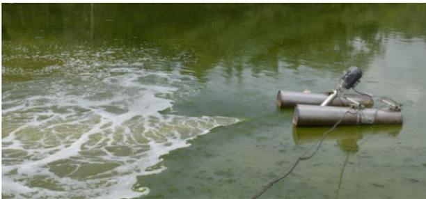
We are also assisting the San Isidro wastewater facility in Costa Rica by investigating ways to achieve more mixing and aeration in their large lagoon system. A good option is solar powered mixer/aerators, as the plant cannot take on much more power load and needs a low-maintenance solution. This choice could enhance the operation of the lagoon under the existing electrical service.
